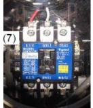
**Electric Contactor under** 240V, 50A cannot ignite R32.
